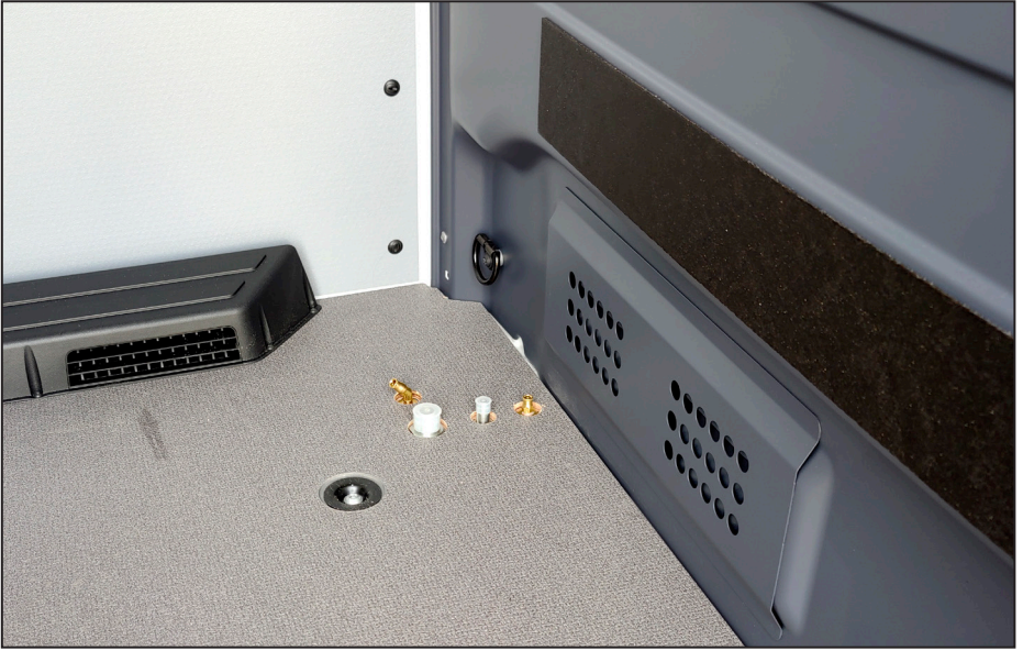
Figure 24 — Bulkhead fittings installed (interior view) (some applications may not include subfloor)
