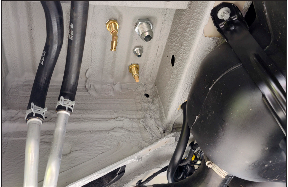
Figure 25 — Bulkhead fittings installed (exterior view)
