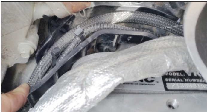
Figure 28 — Installing the cable tray (V300011 compressor shown)
