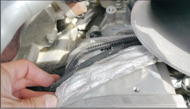
Figure 26 — Installing the cable tray (V300011 compressor shown)
